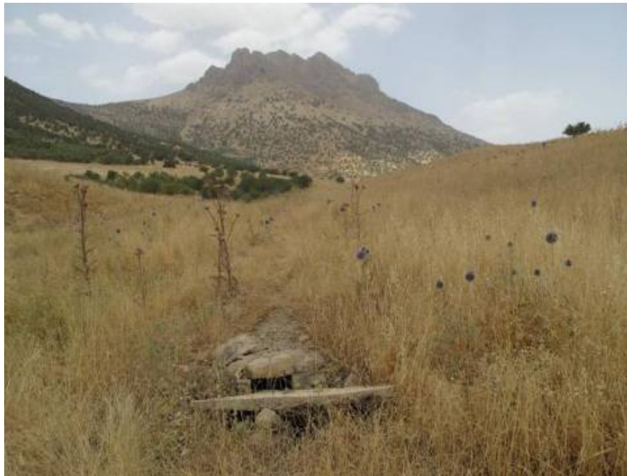
Figure 2. Cut-and-cover section of canal at the outflow of a karez at Basak. (Photo by Dale Lightfoot)
