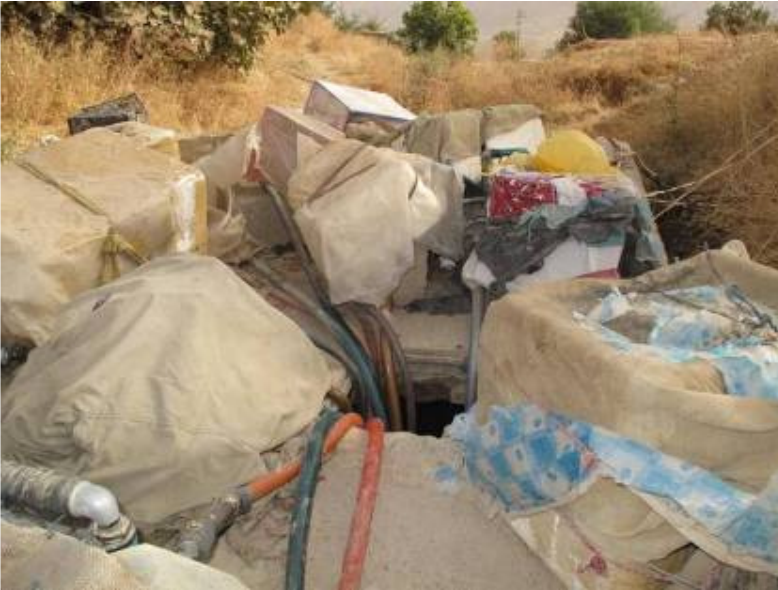
Figure 11. Household pumps drawing from the manjal well (last well before exit) of the Karamuchak karez. (Photo by Dale Lightfoot)
