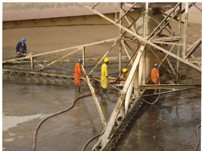
Ref. photo No. C5.1 Clarifier I, cleaning & sludge removing.
