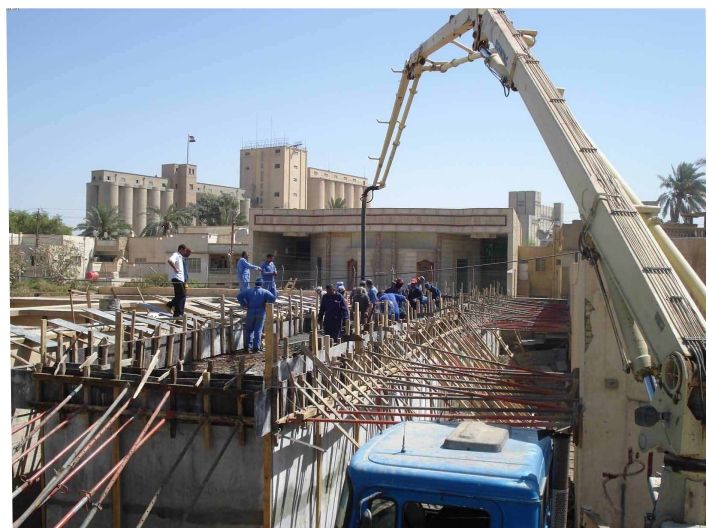
New water tank, roof pouring
