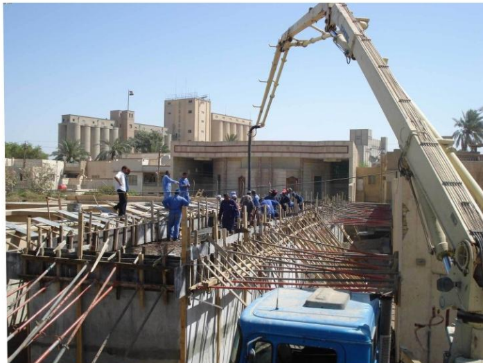
New water tank, roof pouring
