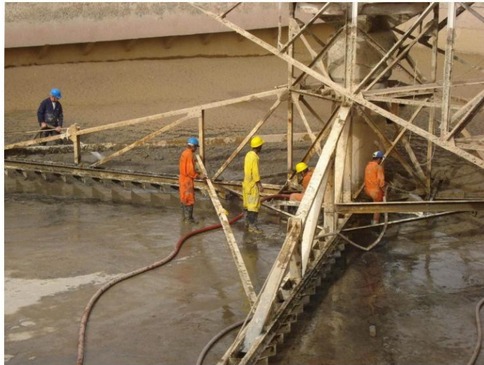
Ref. photo No. C5.1 Clarifier 1, cleaning & sludge removing.
