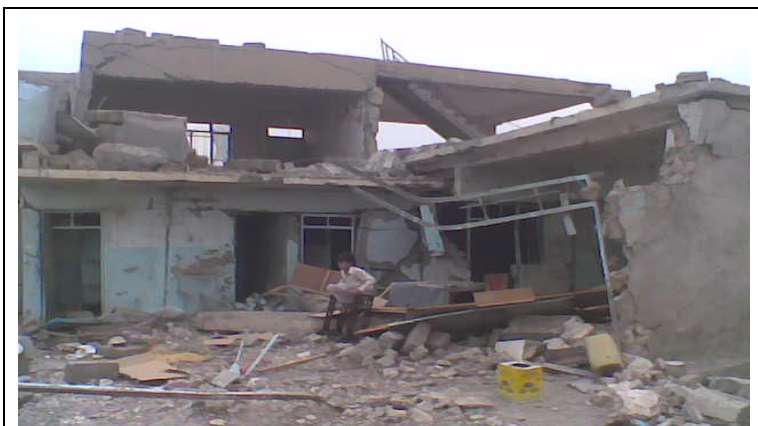
One of the many damaged houses in Shrekhan Sufla. Source IOM
