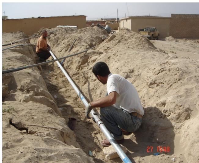
Men from Taq-Harb Village installing water lines.
