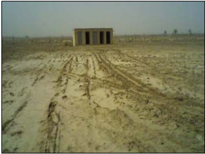
Camp bath and toilet facilities.
